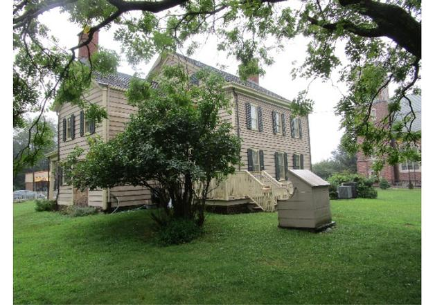
Rain gardens can be installed in the turfgrass areas around the building to capture, treat, and infiltrate stormwater runoff from the roof by redirecting the downspouts into the gardens. A preliminary soil assessment suggests that more soil testing would be required before determining the soil's suitability for green infrastructure.
