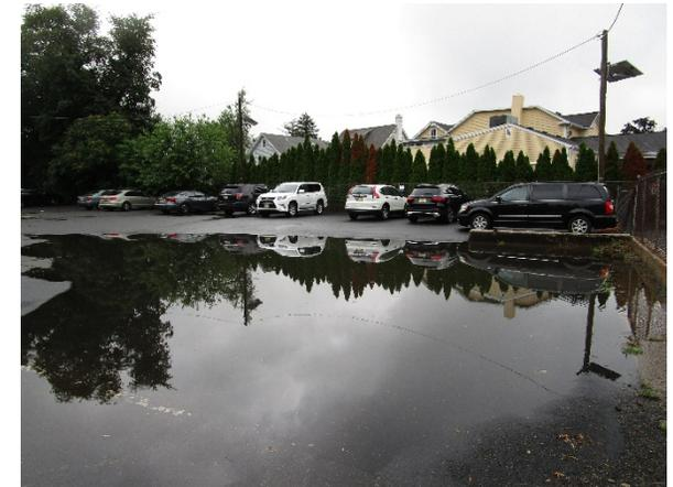
Parking spaces in the parking lot at the back of the building can be converted to porous pavement to capture and infiltrate stormwater runoff from the parking lot. Porous pavement can also help drain the large pooling area of the parking lot. A preliminary soil assessment suggests that the soils have suitable drainage characteristics for green infrastructure.
